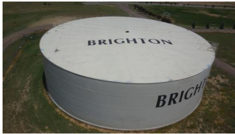
3,000,000 gallon ground reservoir
