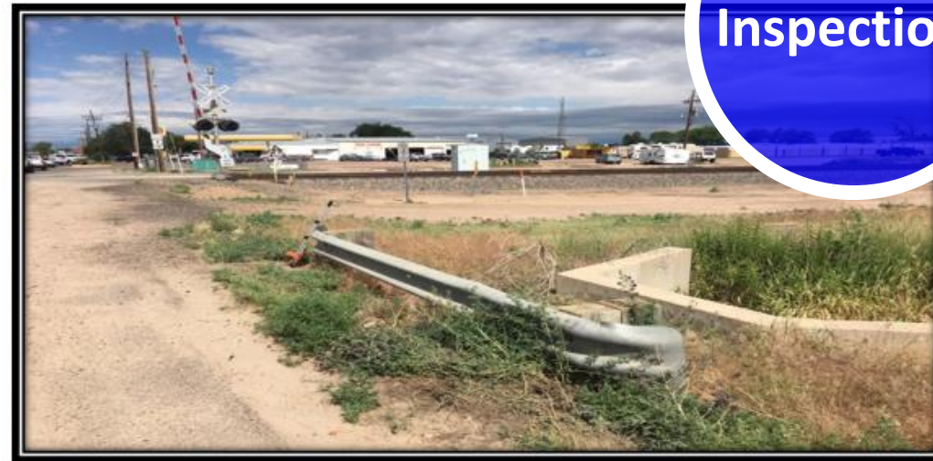
FIGURE 22: VIEWING GUARDRAIL FROM THE EAST IN THE WESTBOUND DIRECTION APPROACHING MAIN STREET (CR27)
