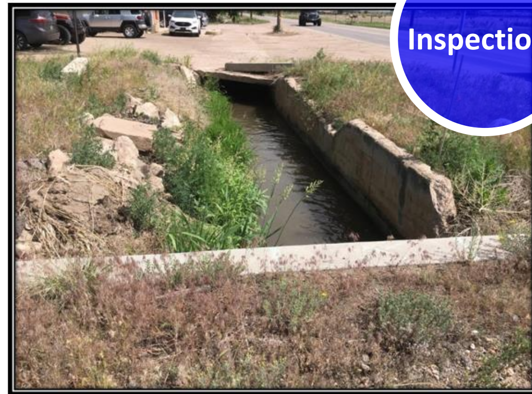
FIGURE 13: VIEWING NORTH ON THE WESTBOUND SIDE OF THE DITCH
