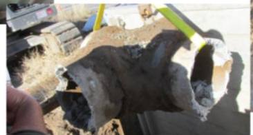
Asbestos pipe removal
