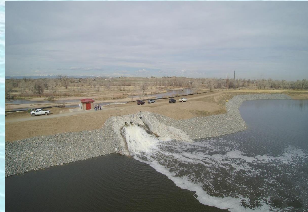
Erger's Pond construction complete and Filled during summer 2019
