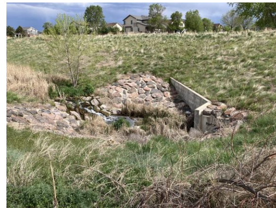
South Outfall Phase II Culverts Flood Control
