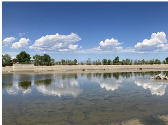
Lutz Reservoir Sustainable Irrigation System
