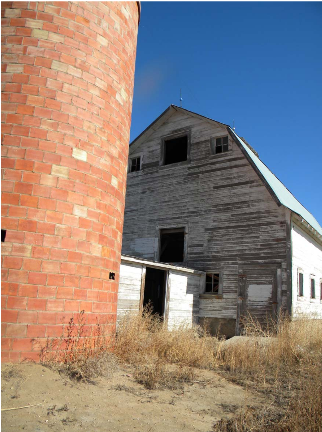
Wood frame extension on west end of barn attached to tile block silo, Foley Farm (5AM.889), view looking northeast.
