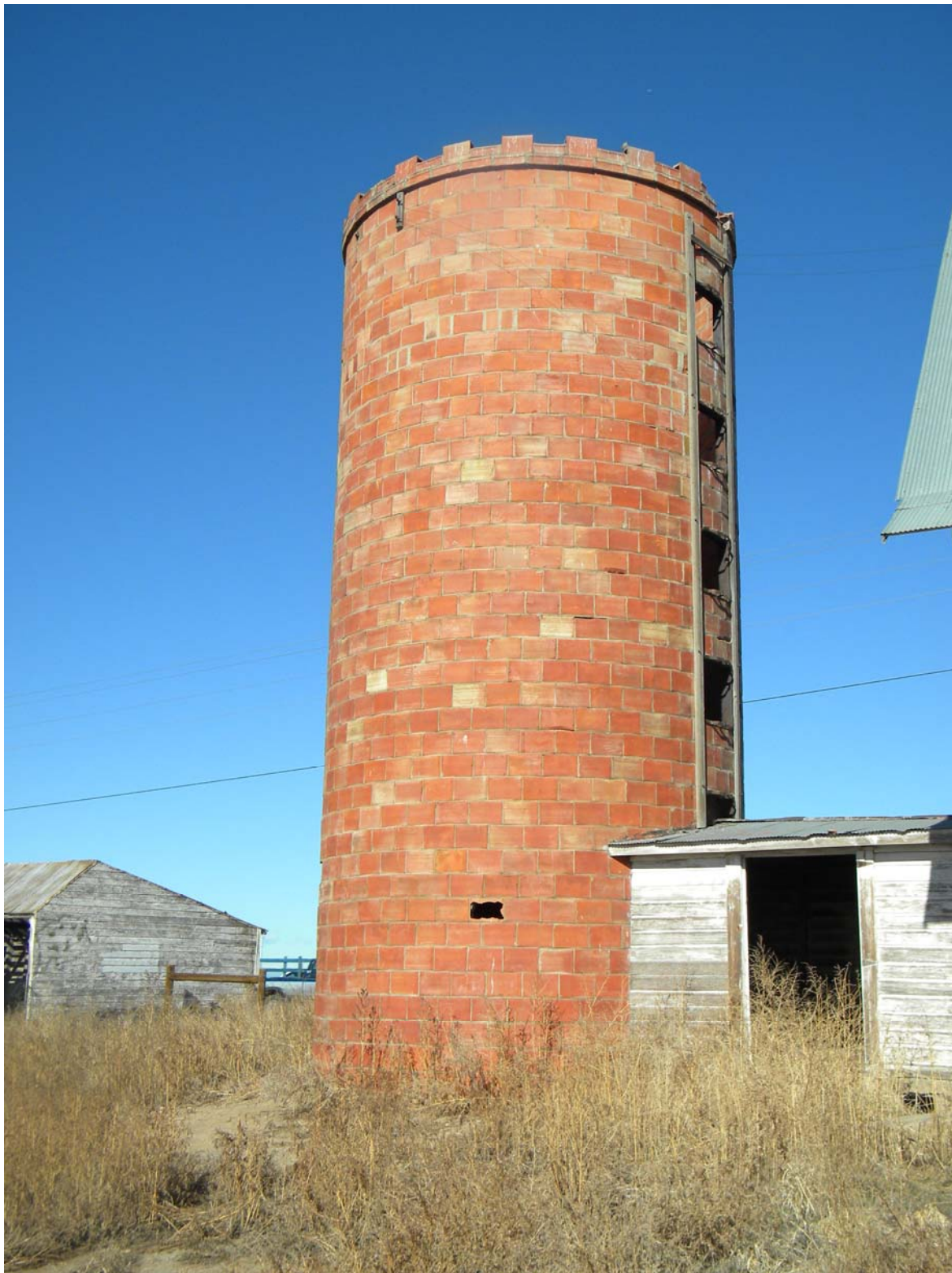
Tile block silo located near west end of barn on Foley Farm (5AM.889), view looking northwest.
