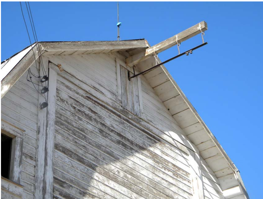
Hay loft lifting apparatus, beneath east gable of barn on Foley Farm (5AM.588).
