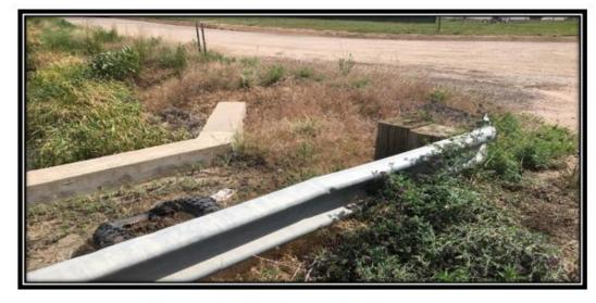
FIGURE 23: MINOR BEND TO GUARDRAIL IN THE WESTBOUND SIDE
