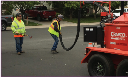
Crack Seal Repair
