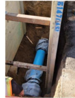
New PVC replacing asbestos tee
