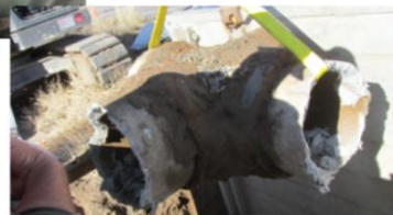
Asbestos pipe removal
