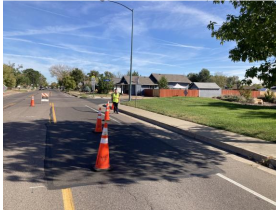
Core City Phase III Waterline Replacement
