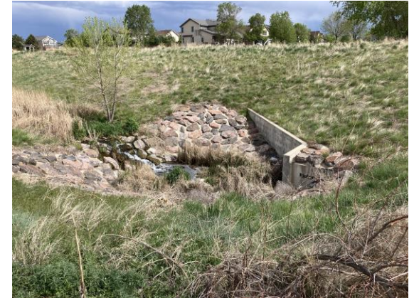
South Outfall Phase II Culverts Flood Control
