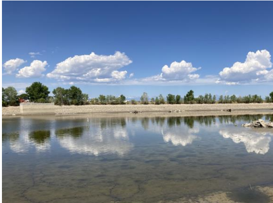
Lutz Reservoir Sustainable Irrigation System
