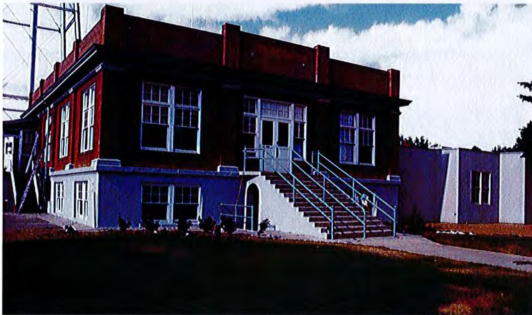
1986 photos of the structure during and after the senior center addition
