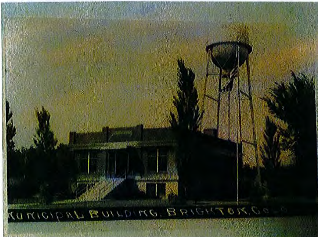
Demonstrates parapet renovations and the water tower on site. Dated between 1939 - 1986
