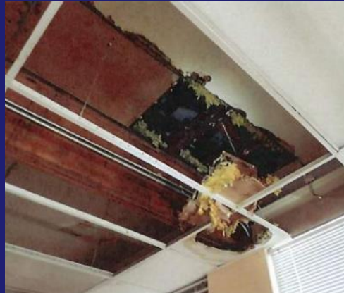
Roof framing at original building
