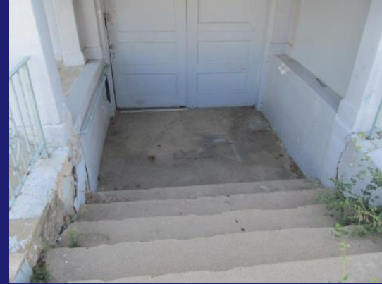
West Area Well – No area drain (right photo)
