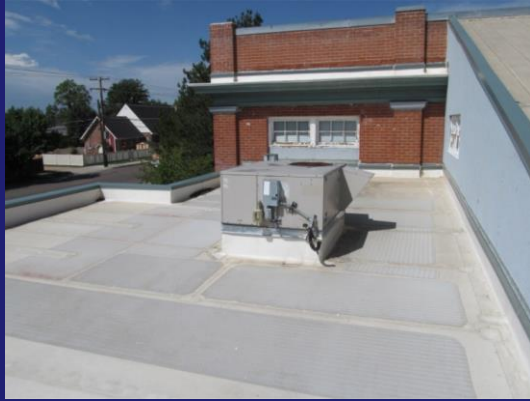
Roof of Addition – Replaced in 2013 (left photo)
