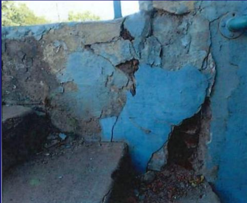
Base of north column at base
