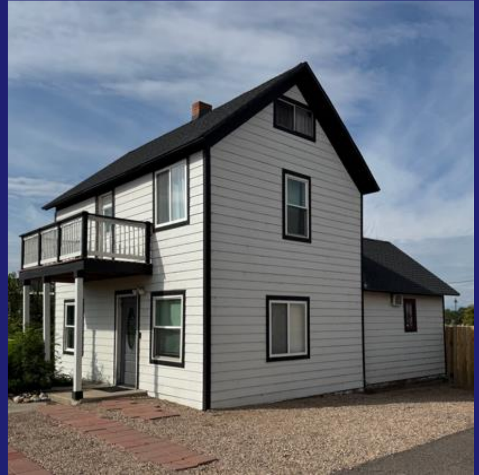
Oblique of 319 South Main Street
