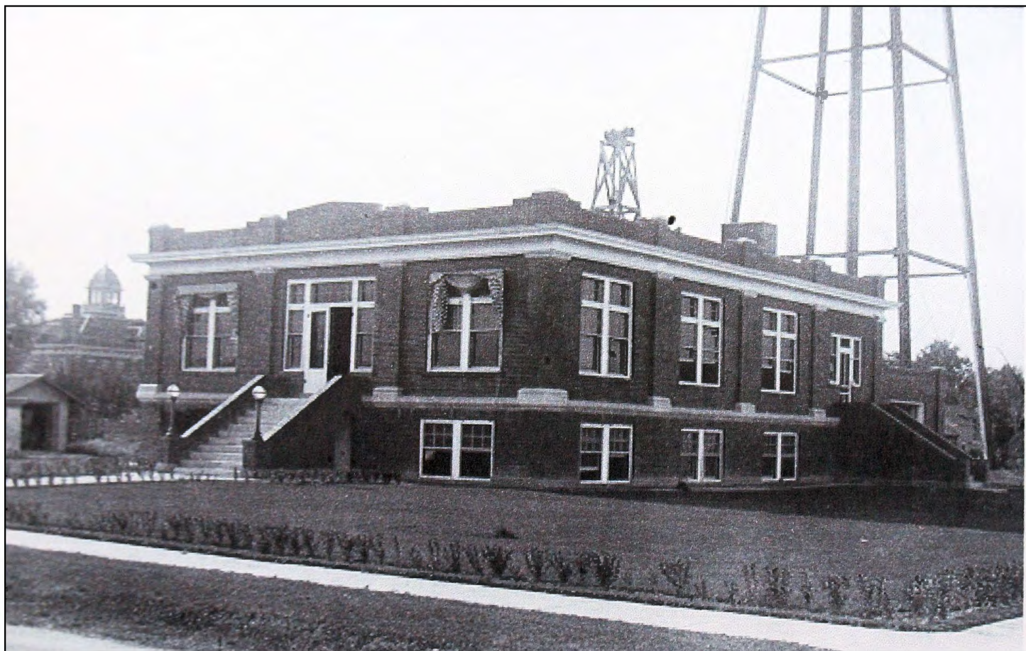
Figure 4. Historic view of Brighton City Hall/waterworks building, with water tower at the rear (no longer extant). Source: Pat Reither collection.
