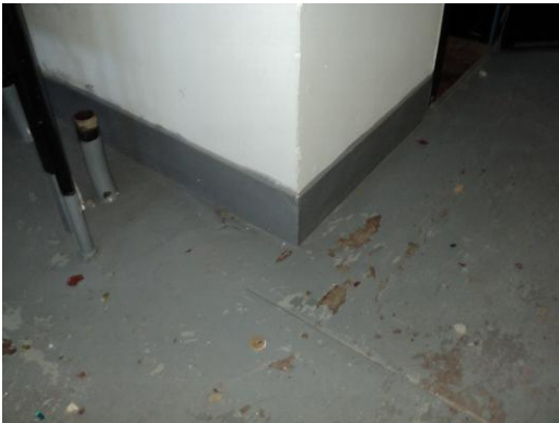
#12 Boiler Room Baseboard
