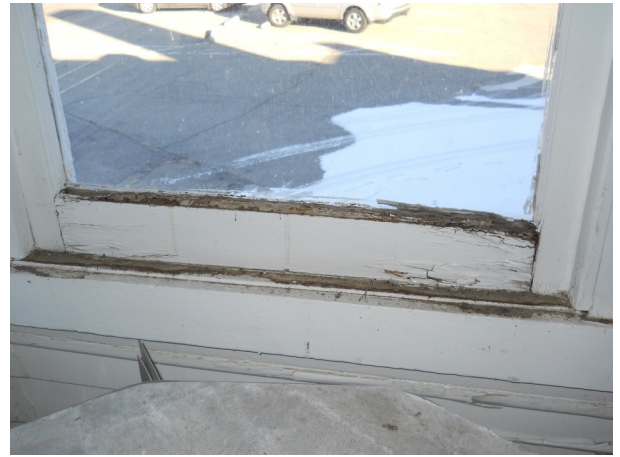
Window at west porch
