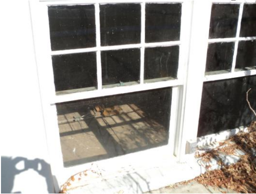
#13 Exterior Side 2 Window Components
