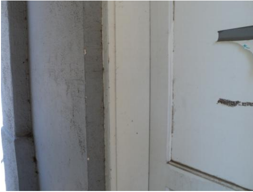
#13 Exterior Side 2 Lower Door
