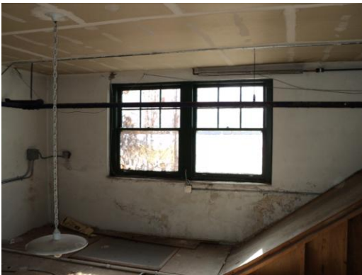
#12 Boiler Room Wall 2 Window
