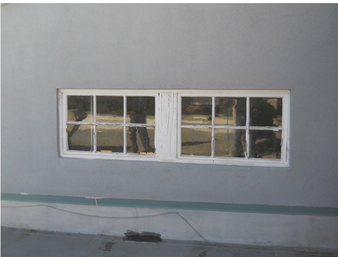
Window on side of shed roof at 1986 addition
