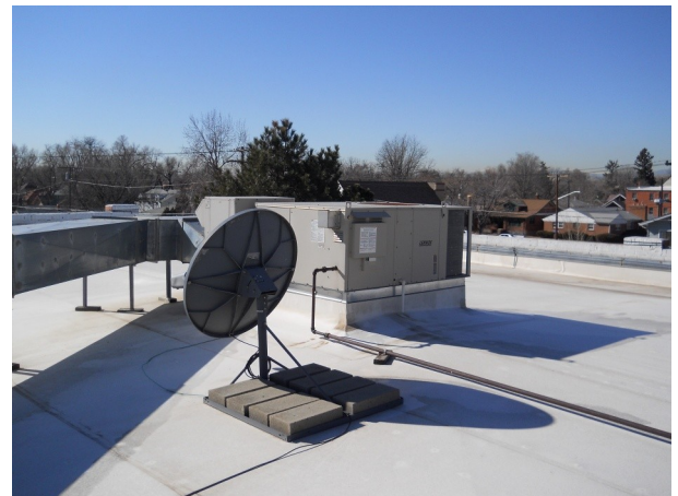
Roof at original building
