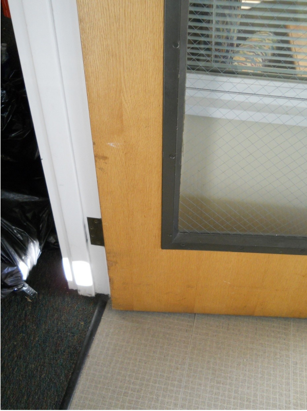
East entry vestibule door
