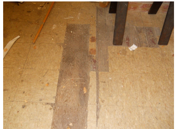
VCT floor at basement entry
