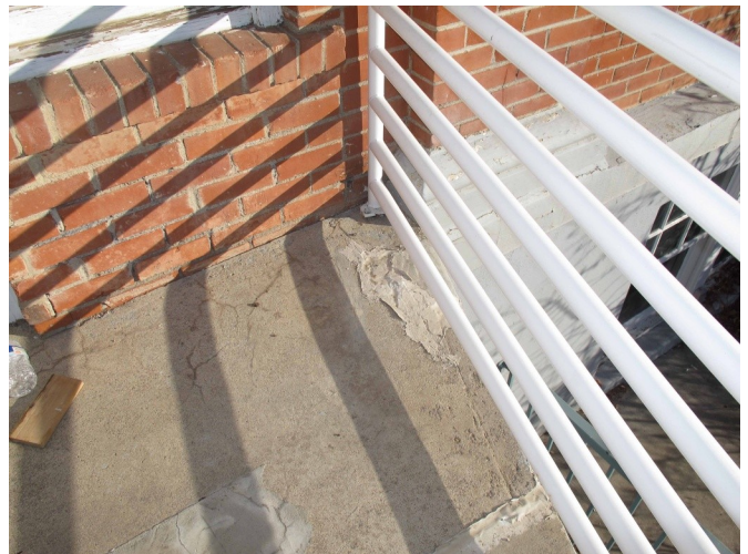
Concrete deterioration and cracking at the south entry stair landing
