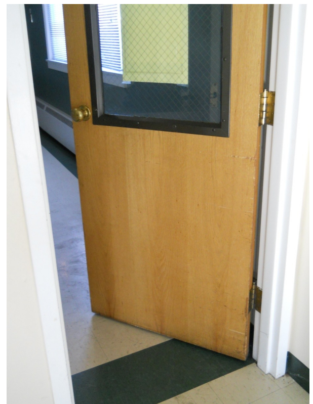
Door between kitchen and dining room
