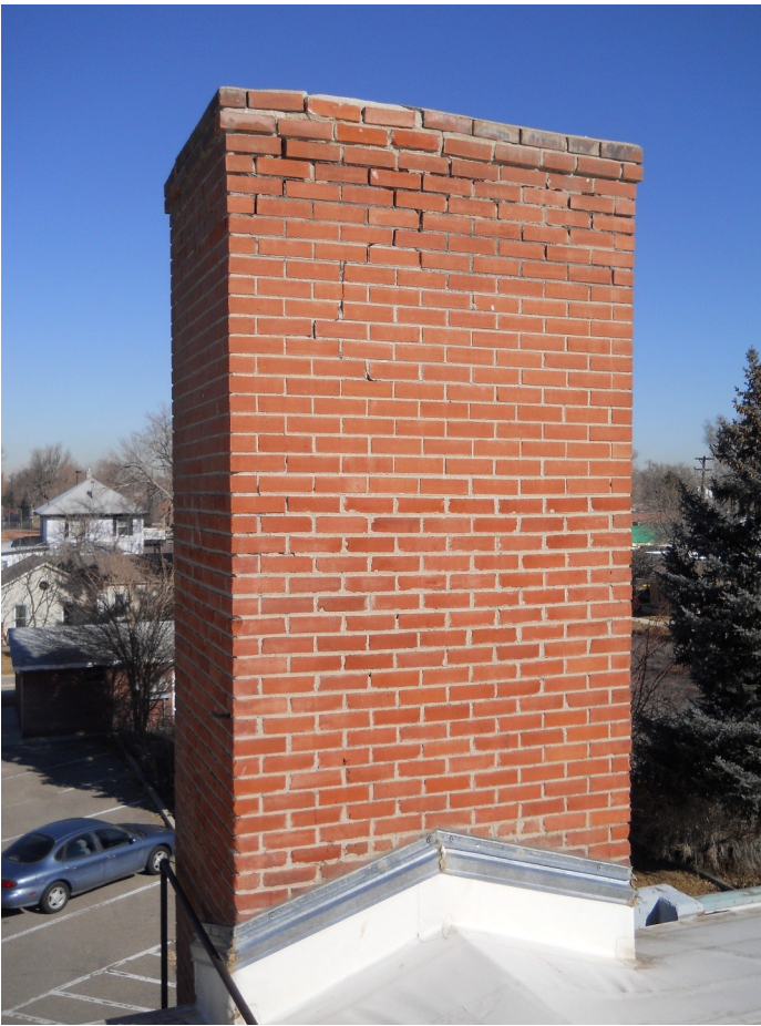
Chimney at original building
