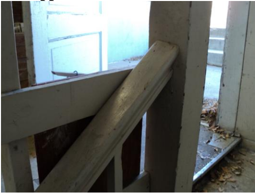
#10 Upper Basement Handrail
