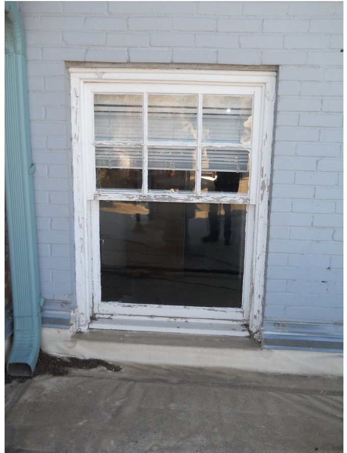
Upper level window at above north wing roof
