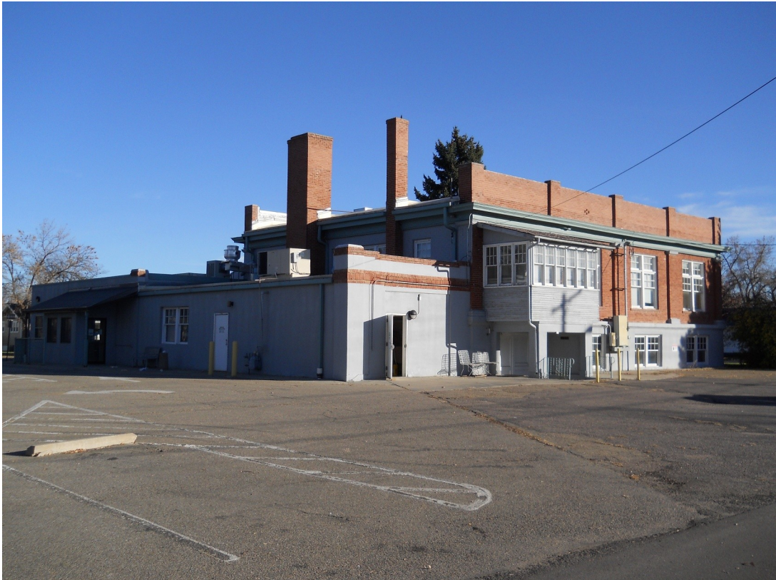
North and West Elevations
