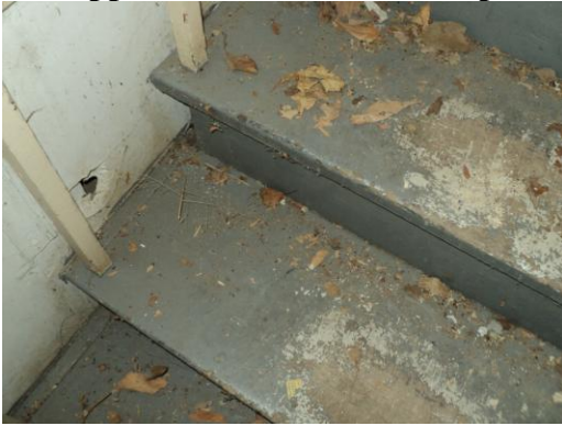
#10 Upper Basement Stair Components
