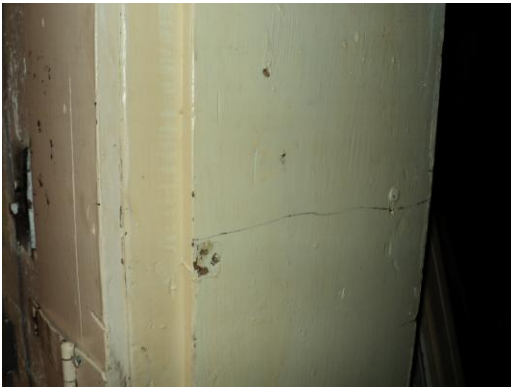
#11 Lower Basement Wall 1 Door Jamb
