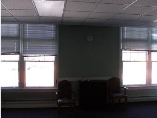
#2 Activity Room Wall 3
