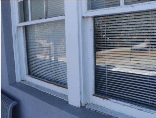
#16 Exterior Side 4 Window Components
