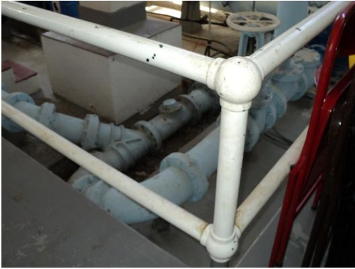
#12 Boiler Room Handrail
