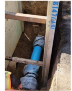
New PVC replacing asbestos tee
