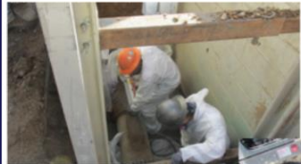
Asbestos pipe removal
