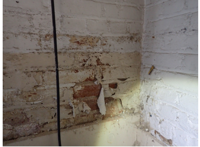
Brick in basement
