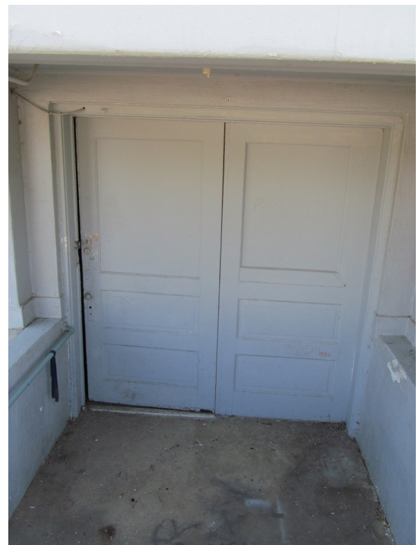
West entry to basement
