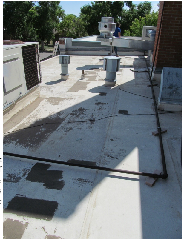
Roof of north addition
