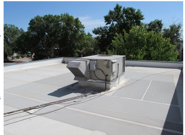
North roof at 1986 addition
