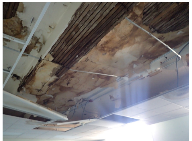
Upper level ceiling at original building
