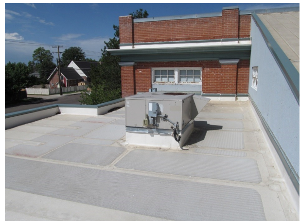
South roof at 1986 addition
