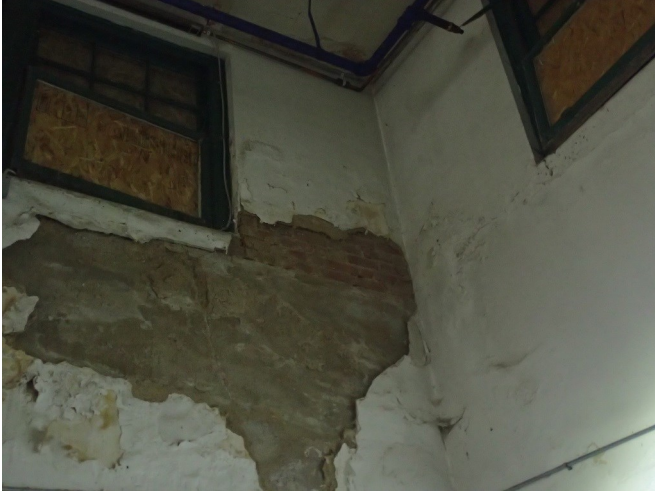
Parge coat at basement wall
