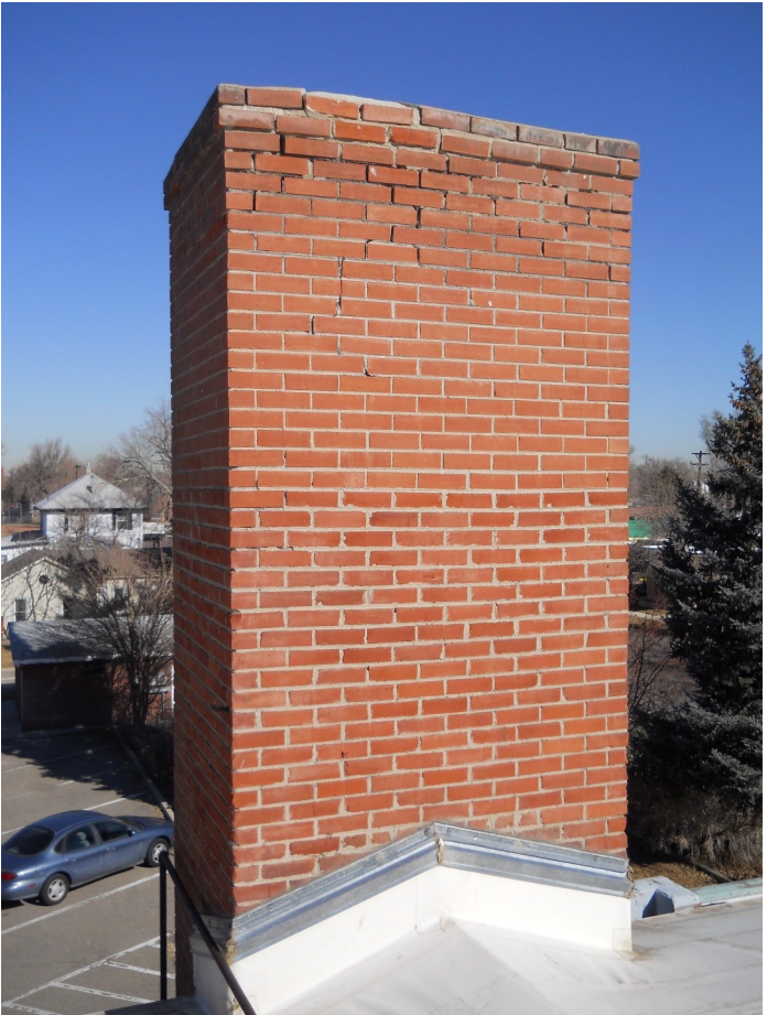
Chimney at original building
