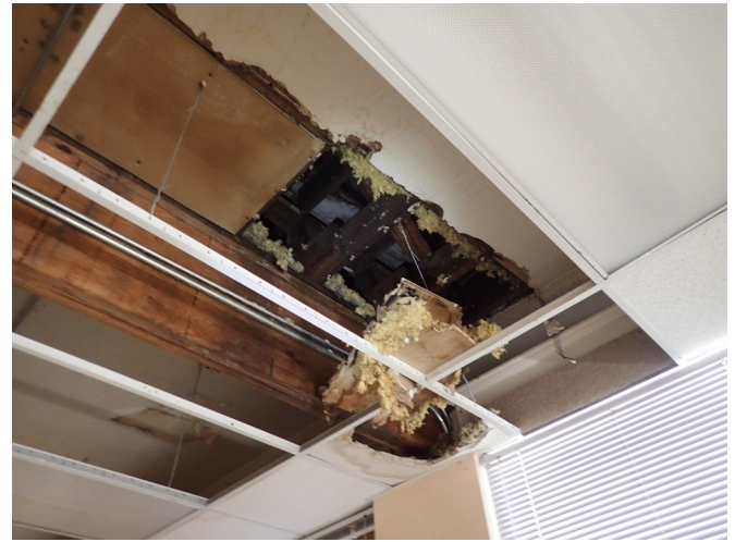
Roof framing at original building
