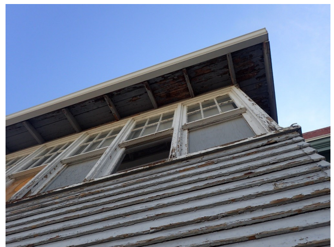
Wood framing at enclosed balcony
