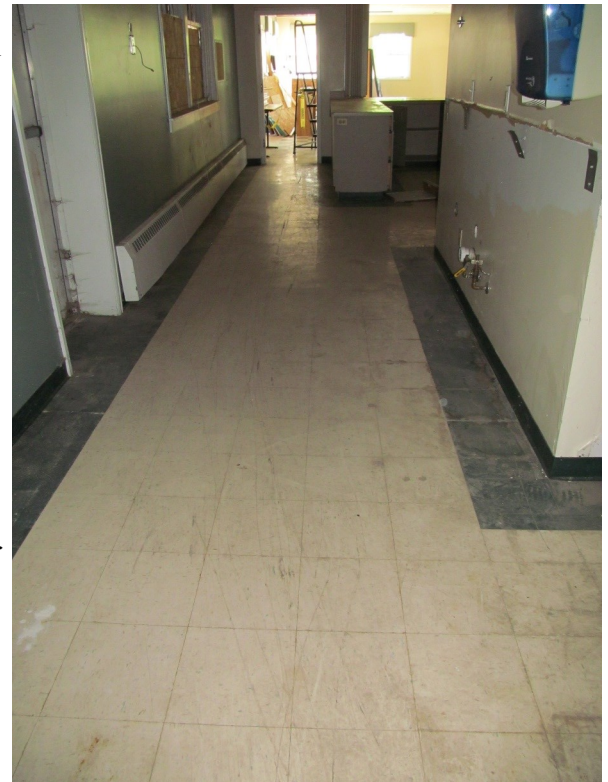
VCT flooring at kitchen
