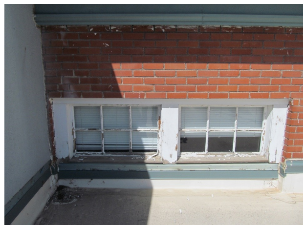
Windows at upper level
