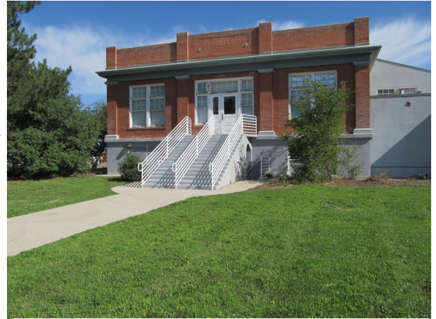
South side of building
