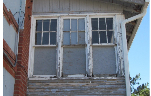
Windows at west porch
