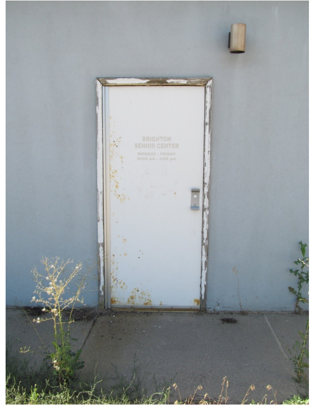
North kitchen entry door
