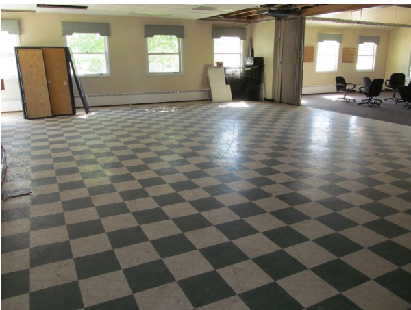
VCT flooring at dining room
