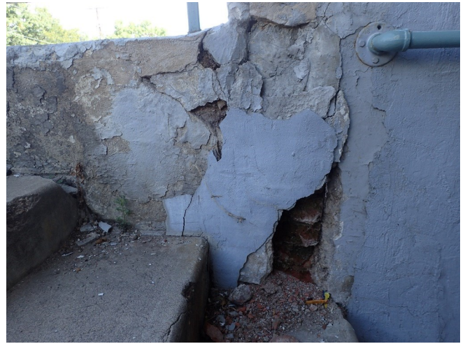
Base of north column at balcony
