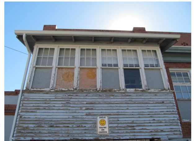
Windows at west porch
