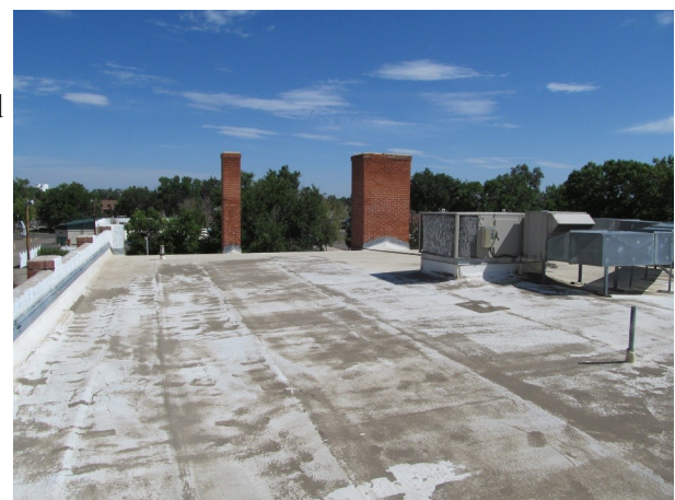
Roof at original building
