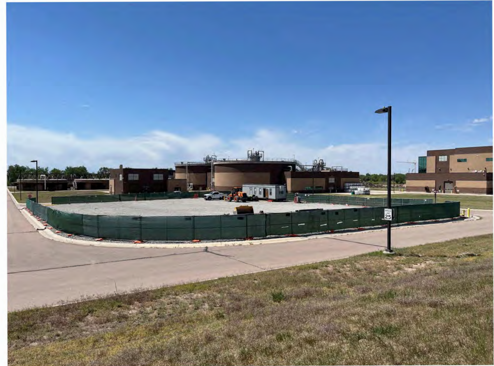
Construction Staging Area with screening fence around perimeter
